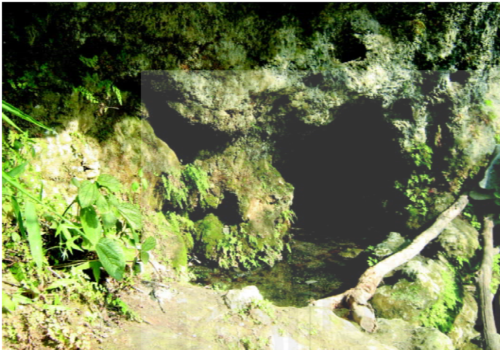
Fig. 7.17: Subsurface water channels are visible at the left bringing water in the main channel at Sahastradhara, Dehradun, Uttarakhand.
