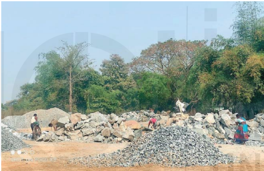
Fig. 7.18: Crushing of Granitic Rocks by Humans for use as Construction Materials.
