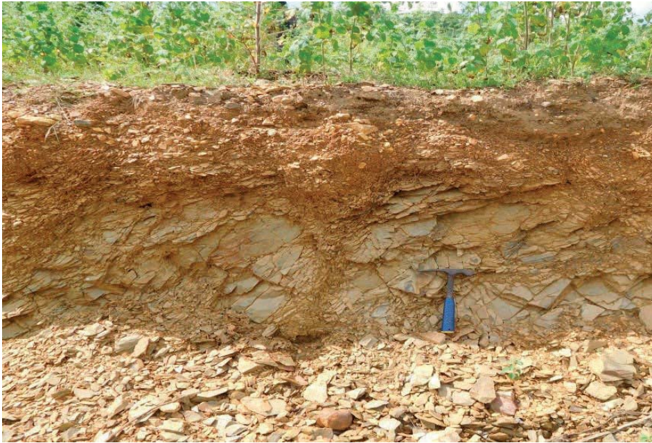
Fig. 7.5: Granular Disintegration of Rocks (Pakhal Super Group).
