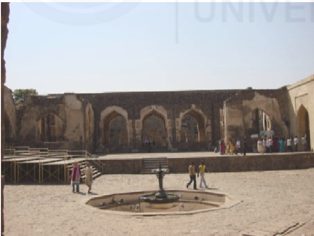
Figure 23.2: The central area of the Golconda Fort, with the zenana in the background, and a fountain in the central courtyard. Photograph by Radhika Seshan
