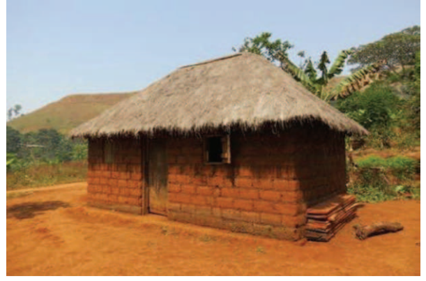
Fig.14.5: Brick and Thatch House.
