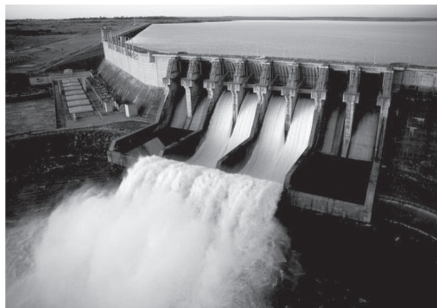
Fig. 10.4: A Hydro Power Project with Water Discharging Sluice Gates.
