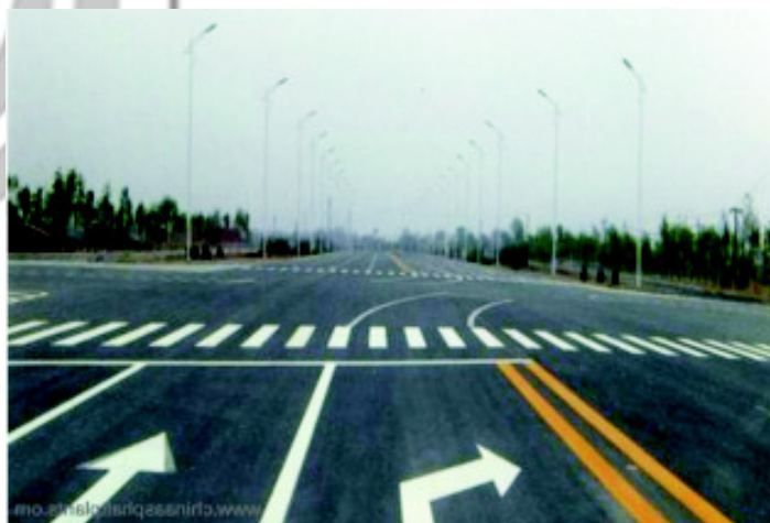
Road surface markings to differentiate right and Straight Traffic Movements.
